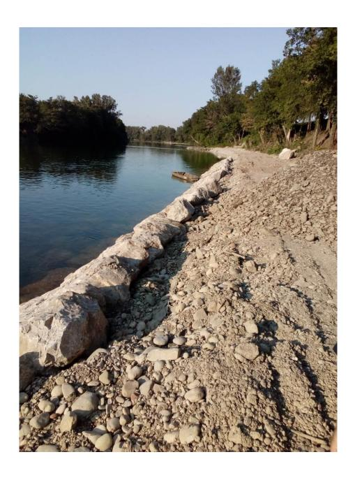
Photo taken during construction of bank revetments on Vrbas river in previous years, area of Veliko Blasko.
